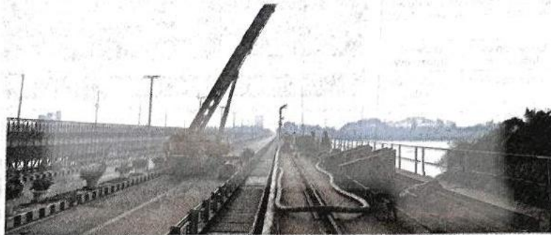
Work being carried out at the barrage last week. Amit Mehra
