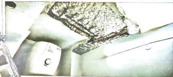
Soon after Gaurav Pandey purchased his first floor flat, a portion of the bathroom ceiling fell.
