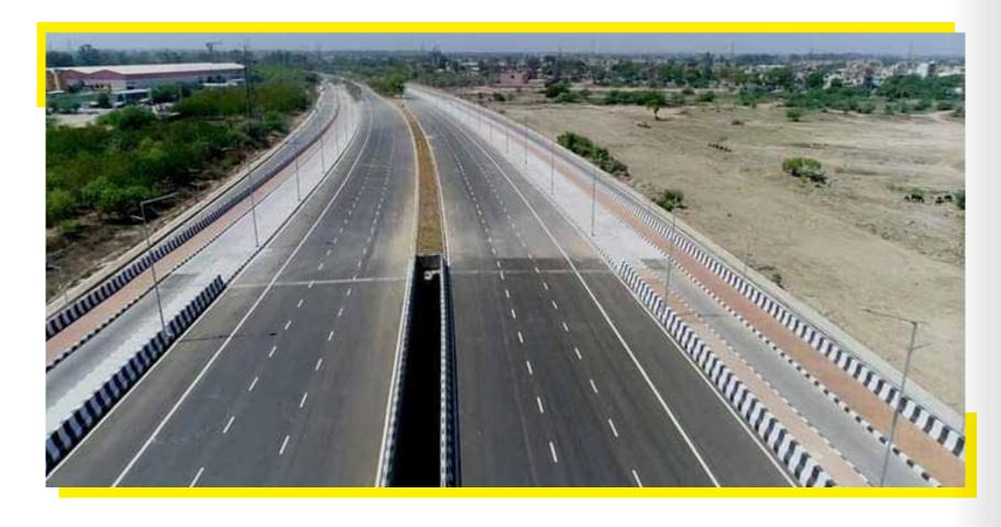
Arrangements have been made for proper drainage and harvesting of Rainwater from the ROB through Rainwater Harvesting Structure.
