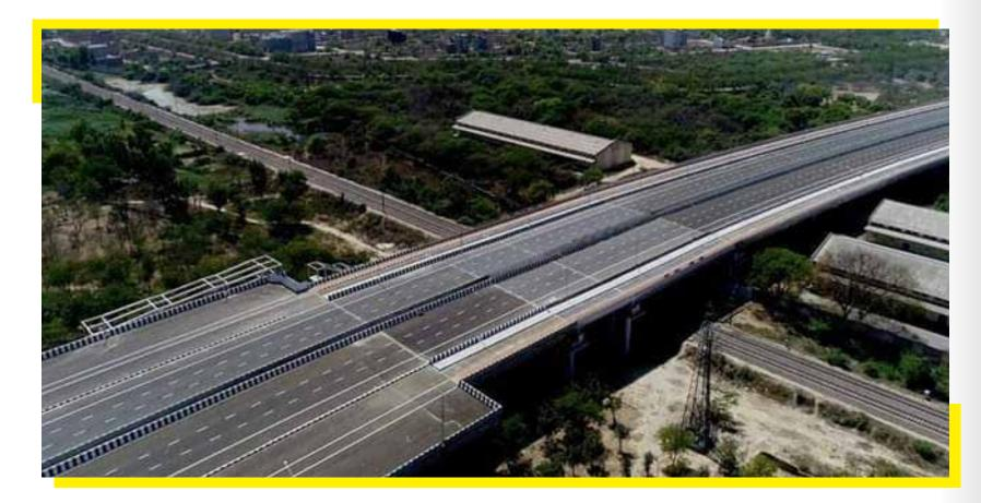
The Road Over Bridge has provision for two separate carriage ways of 25.5 m each, consisting of 3 lane carriage way, dedicated bus lane, cycle track, utility corridor and footpath with patterned colour concrete.
