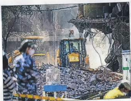
DDA initiated the demolition drive last Friday.
