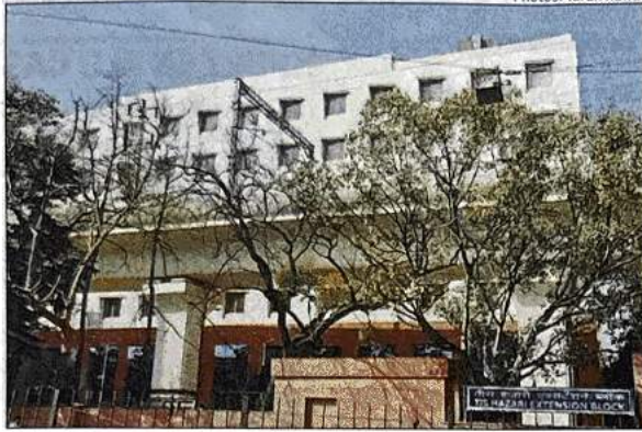
The six-storey extension of Tis Hazari building is nearing completion
